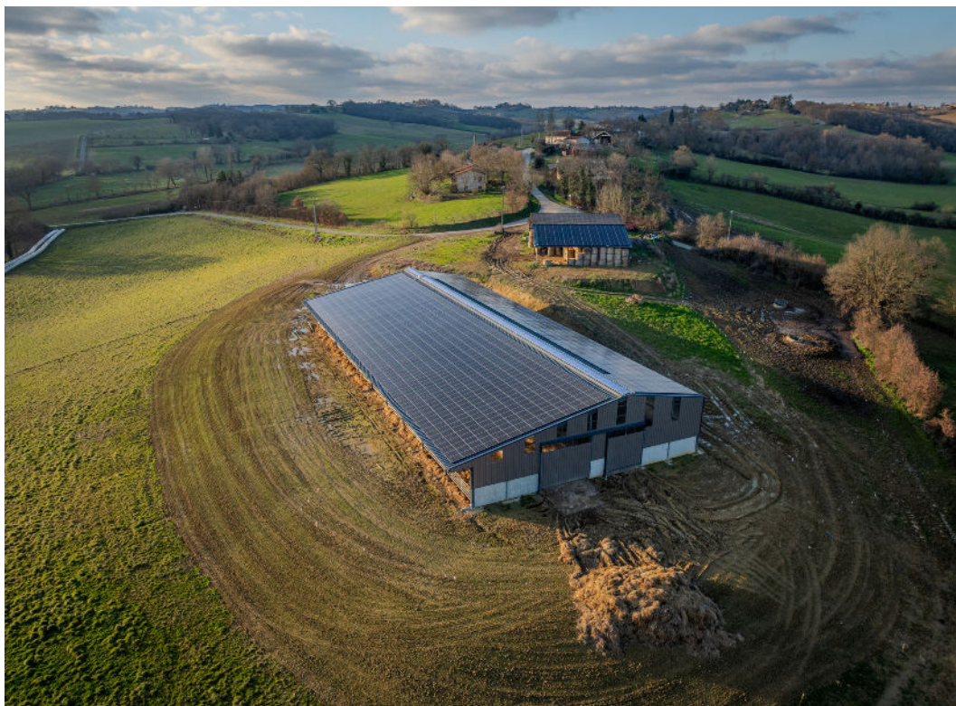
Barn solarisation by Arkolia
