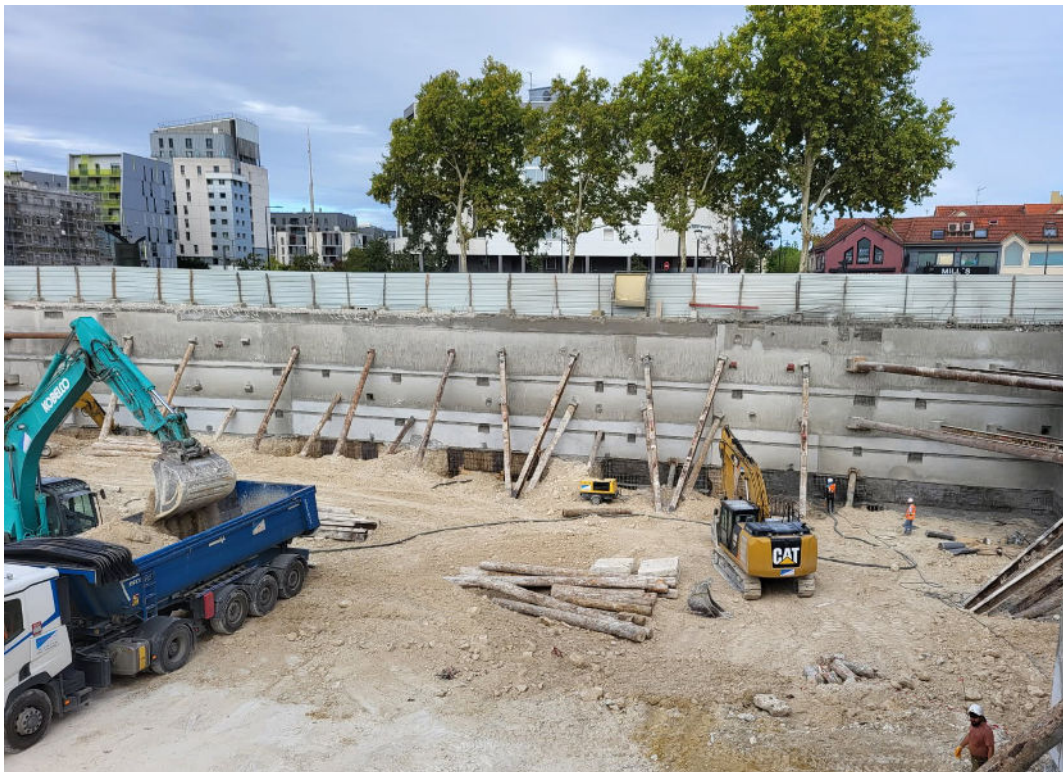
Renovation-operation worksite in Colombes
